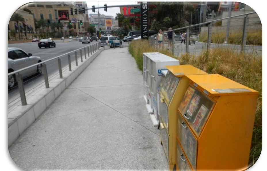
Picture 2.11 – Back of Curb Cable Barrier.
