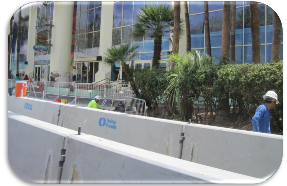
Picture 2.21 – Landscaping/Utility Construction at the Flamingo Hotel/Casino.
