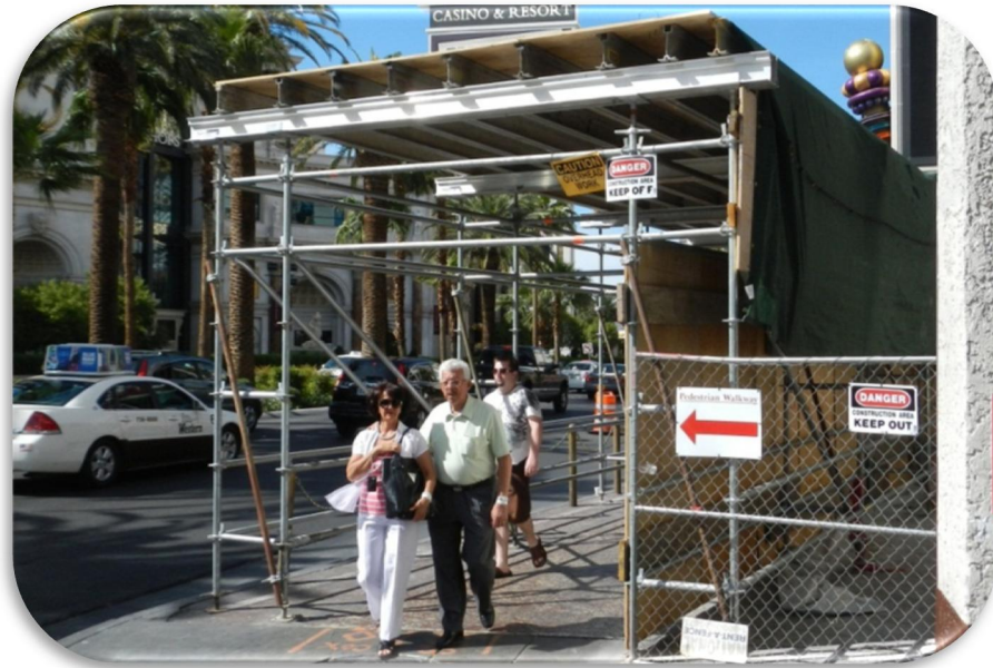
Picture 2.13 – South Entrance to Pedestrian Walkway through Linq Construction.
