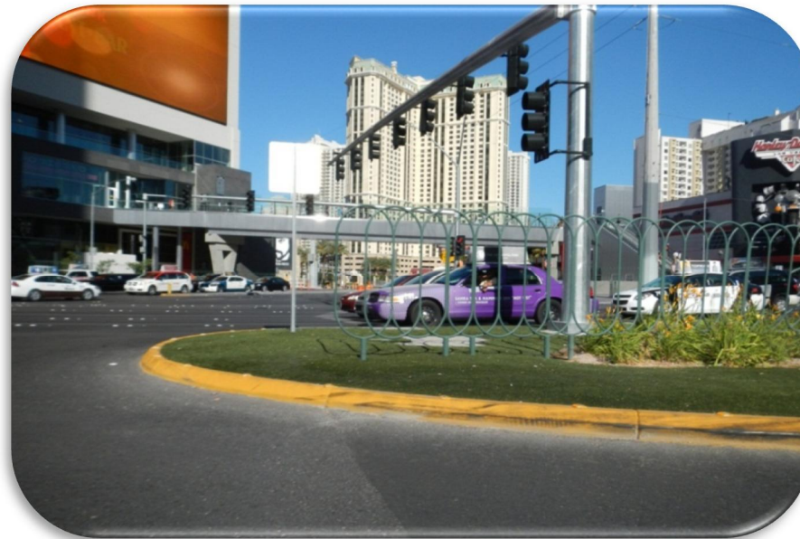
Picture 2.9 – Metal Fence Median Barrier.
