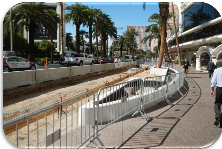
Picture 2.17 – Bus Turnout Construction at Harrah's Hotel/Casino.
