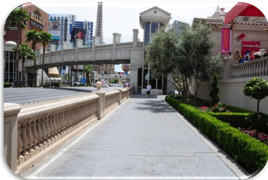
Picture 2.8 – Back of Curb Concrete Wall and Landscape Treatment.
