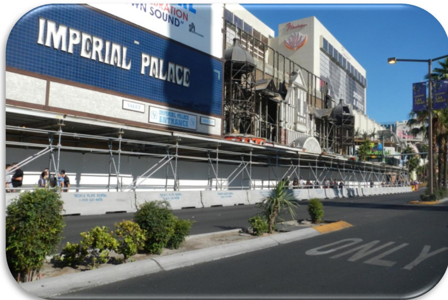
Picture 2.16 – Caesars Linq Construction.
