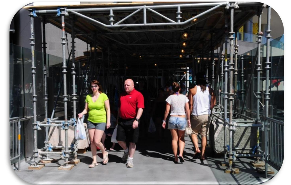
Picture 2.15 – Pedestrian Bridge Detour at Harmon Center from Cosmopolitan Hotel/Casino.
