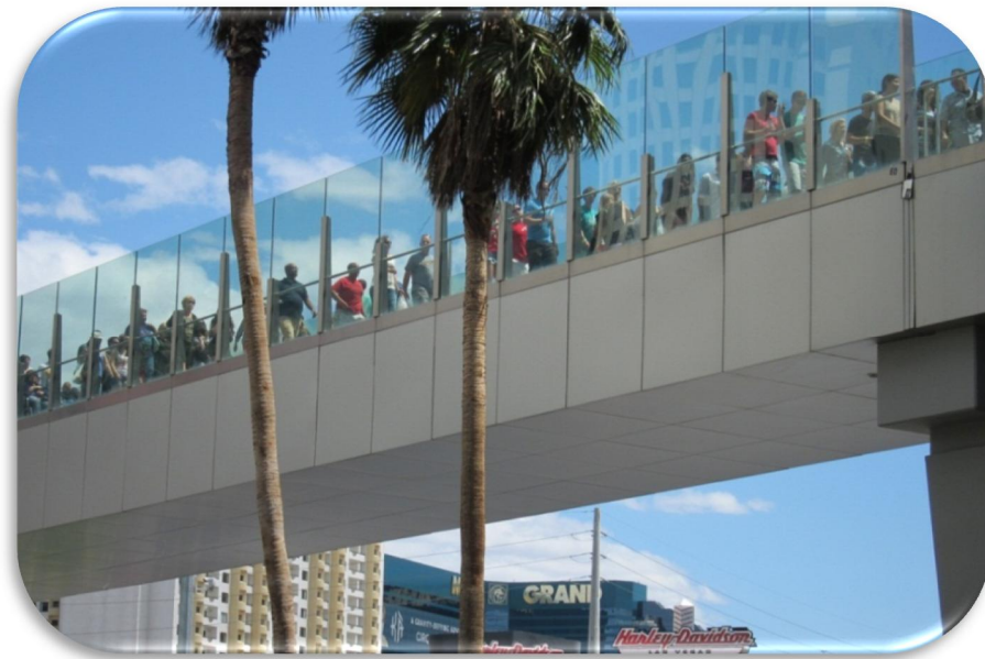
Picture 3.13 – Typical Pedestrian Bridge.
