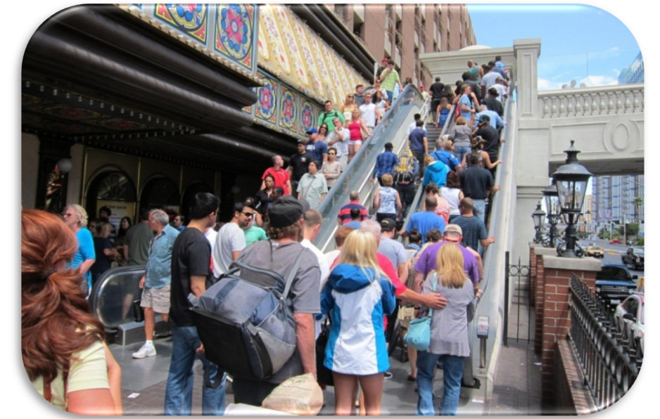
Picture 3.11 – Flamingo Road East Pedestrian Bridge Escalators.
