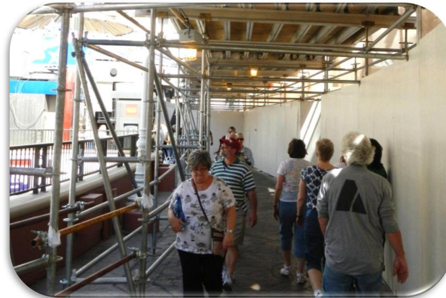
Picture 2.14 – Pedestrian Walkway through Linq Construction.
